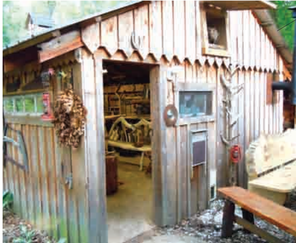
Workshop could be freestanding from both house and garage or be attached to one of them.
