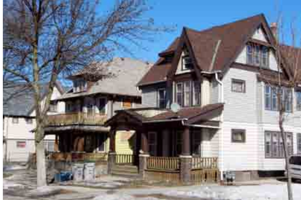
Good Variety at House Scale Image Taken by Mark Roeder
