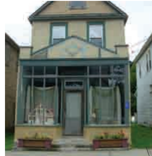
This is a good example of heavily glazed retail space on the first floor with the living space recessed slightly from the front.
