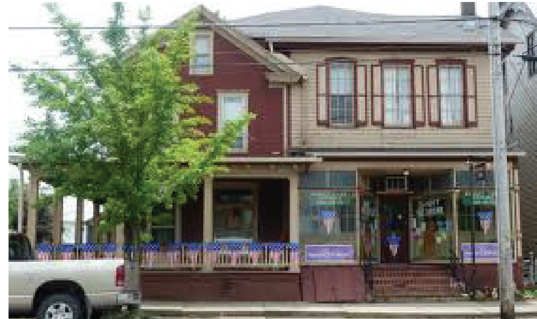
Heavily glazed areas on street level make it easy for owners to advertise their business and have a visual connection to the outside.
