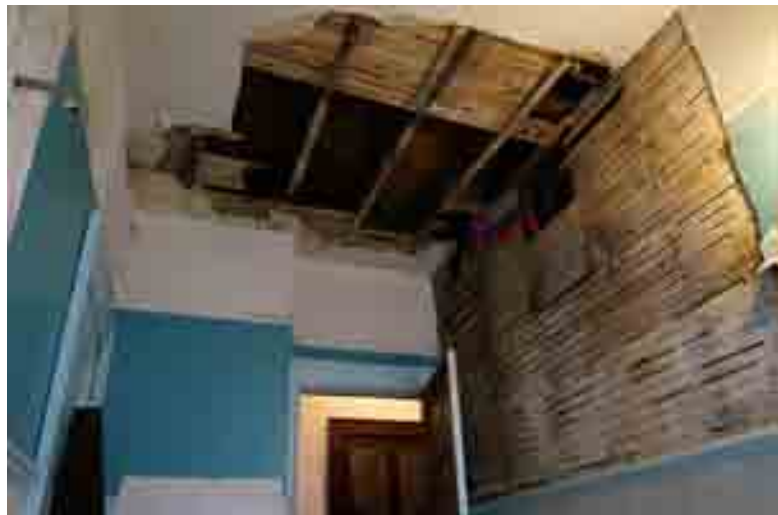
Wall and ceiling renovations.
