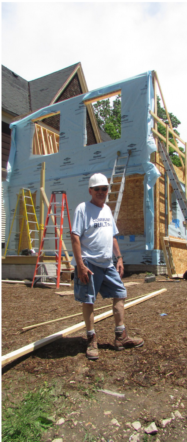
A worker at the Habitat for Humanity work site.
