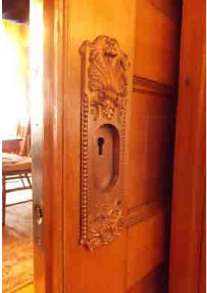
A sliding pocket door in the Frederick Koenig House.
